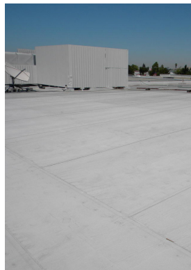
Coating for a low-sloped roof Photo credit: DNG Group
